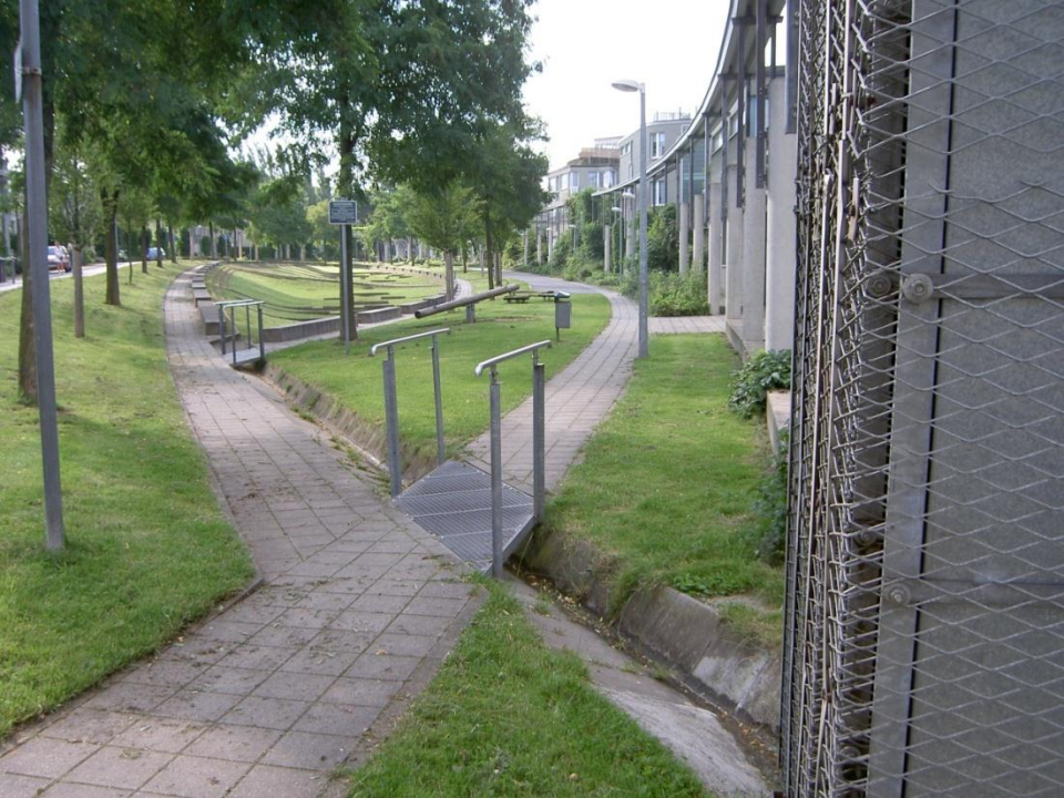
Rain water, Kupperbusch Siedlung, Gelsenkirchen, Germany, Sustainable urban drainage system
