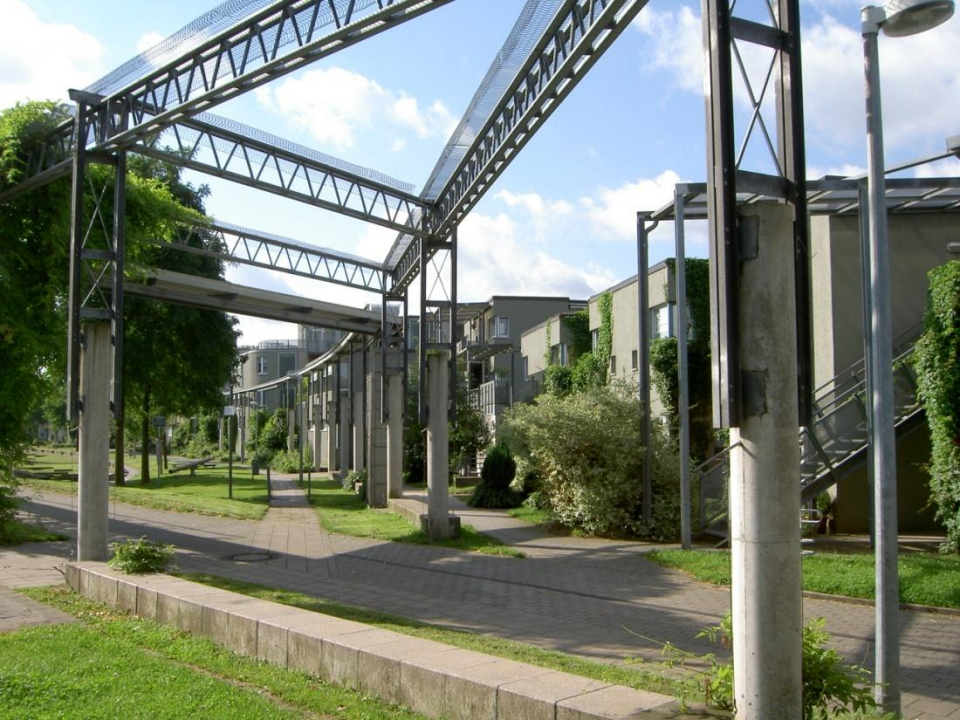
Rain water, Kupperbusch Siedlung, Gelsenkirchen, Germany, Sustainable urban drainage system
