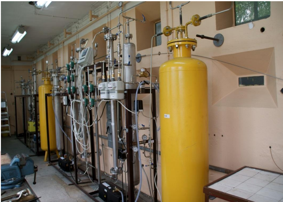
Fig. 1 Installation of biogas purification and enrichment
